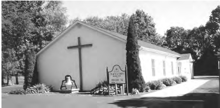
The Bradley, Michigan Local Church dedicated October 1, 1995
